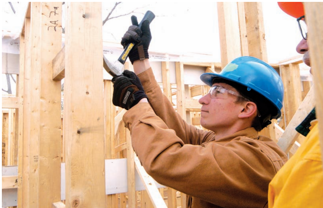
Nicholas Lovasic has been working on a Habitat for Humanity home as part of the Hamilton Catholic school board's home building program. | Photo by Gord Bowes
